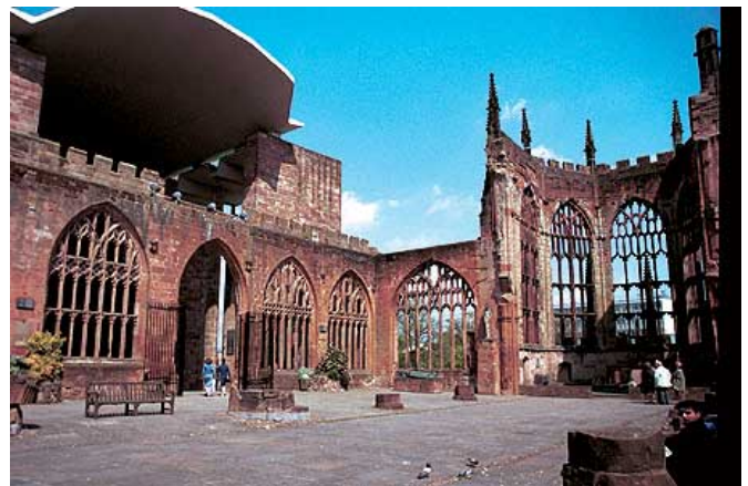
The roof of the new Coventry Cathedral taken from within the ruins of the original building. Photo credit:CoventryPages.net
